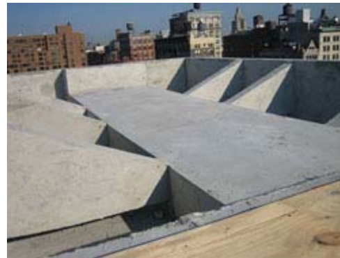
Figure 9 –Penthouse Roof Structure
